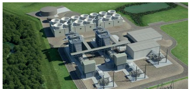
Woodbridge Energy Center | Woodbridge, NJ, USA
